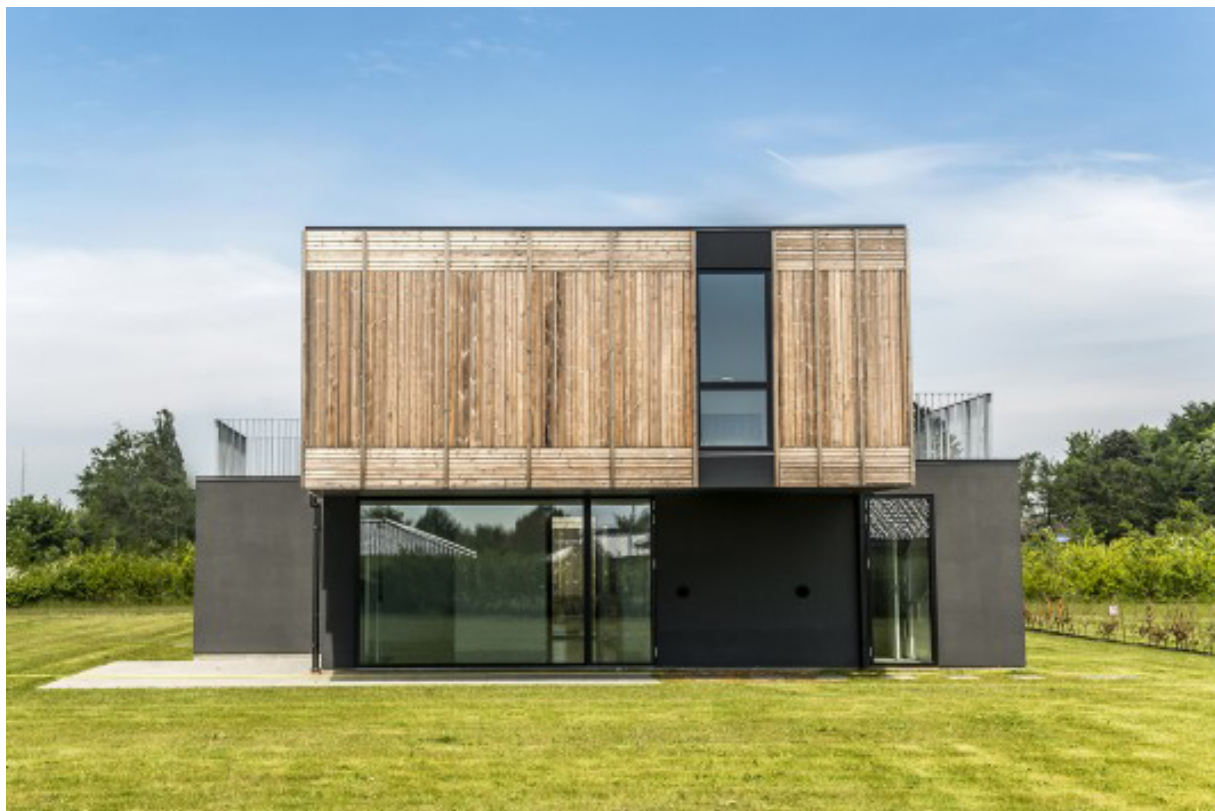
Figure 8 Adaptable house uses concrete in the base for thermal mass, and insulated frame for the upper cantilever (photo: Jesper Ray)
