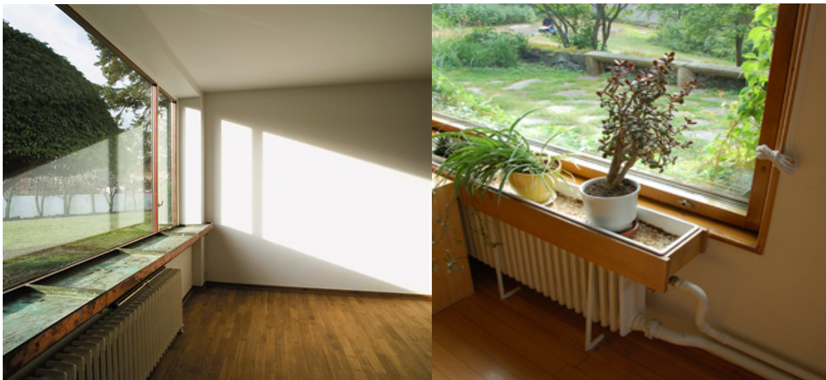
Figure 7 Deep windows and planter boxes above heater with operable window in the Gotfred Rodes House (photo: Per Munkgård Thorsen/ Lars Degnbod)
