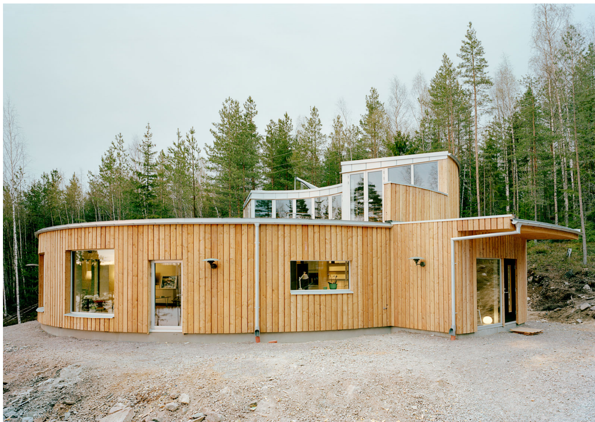
Figure 5 Villa Nyberg exterior; central courtyard brings light and heat into the building, and allows the building to be oriented to the northerly lake views (photo credit: Kjellgren Kaminsky Architecture)
